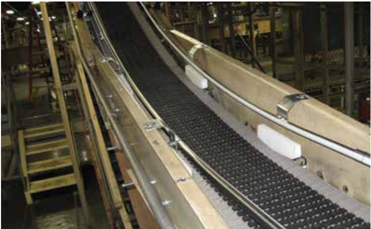
Conveyor with TCF7705 Belt
